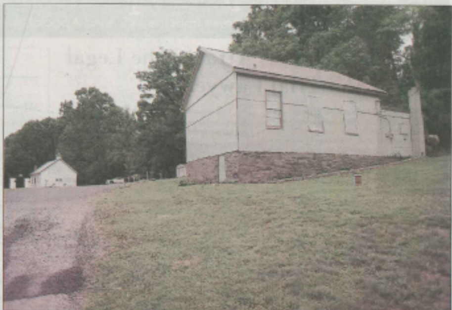
The church (left) is the second built by freed slaves on the Mountain site south of Frederick; the school (right) was built in 1888.
